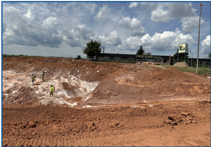
▲ August 2, 2023—Pete Lien & Sons, New Office Expansion in Rapid City, SD. Brett Hunter, Adam Heck, and Dylan Beaver loading Gypsum Shot #1. Note the existing office building approximately 65-feet due west of the nearest loaded blast hole.
